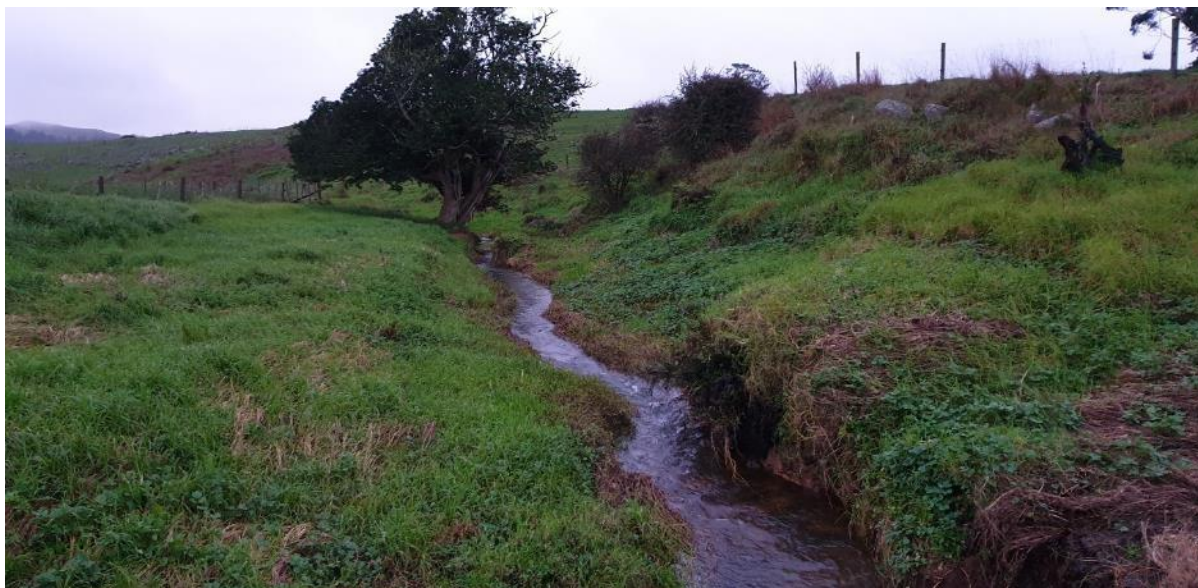
Photo 2: Looking upstream from a culvert crossing approximately 500m downstream of the proposed dam site
